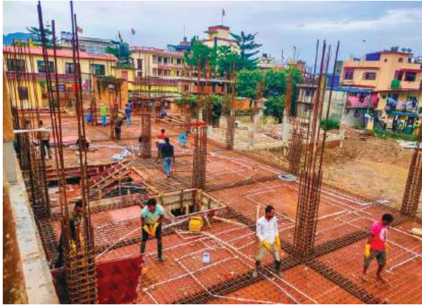
^ Construction Supervision Works
